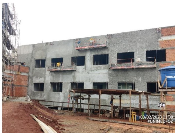
Foto 22 – Reboco – Fachada Principal
